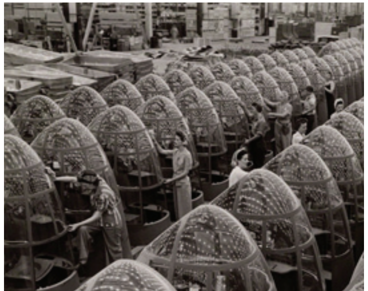
Women aircraft workers finishing transparent bomber noses for fighter and reconnaissance planes at Douglas Aircraft Co. Plant in Long Beach, CA, 1942. Alfred Palmer
